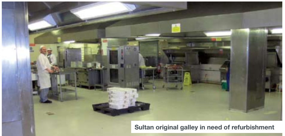
Left: Temporary galley installed at HMS SULTAN for the duration of the works
